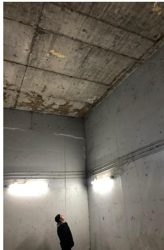
**Honeycombing and poorly made formwork joints**
